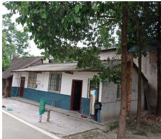
Fig.1 Current Situation of Residential Buildings
